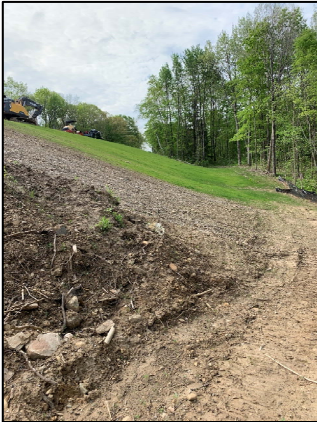
Photo 1 – Stabilized Portion of Fill/Slope
