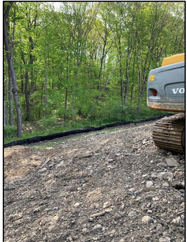
Photo 4 – Single Row of Silt Fence East Side
