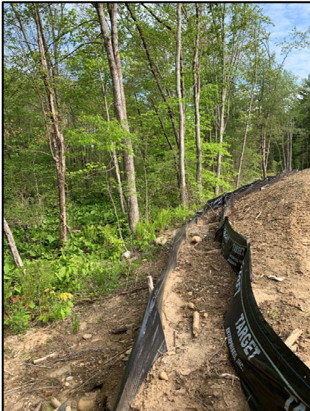
Photo 3 – Double Row of Silt Fence West Side
