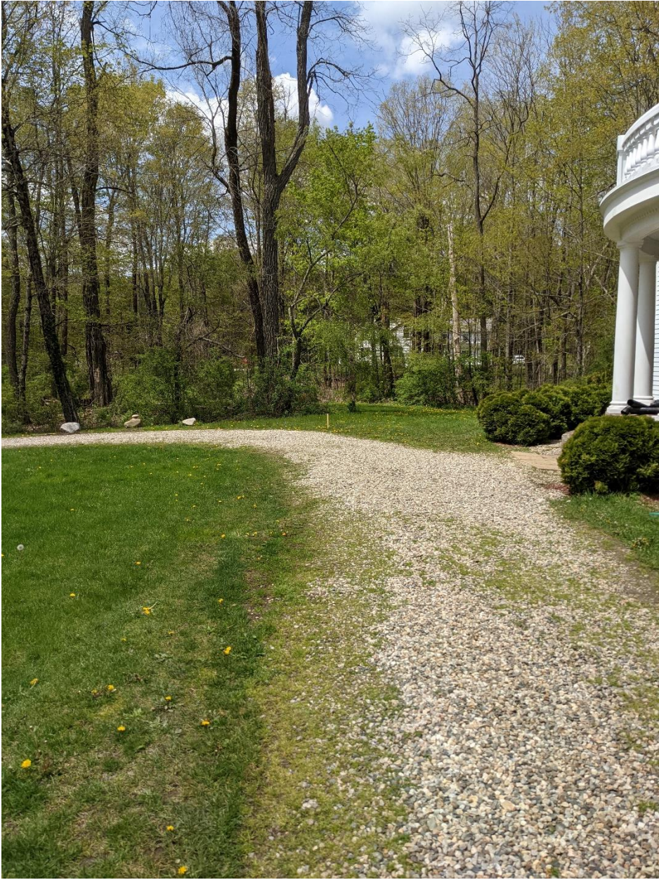
Driveway at front of house. Stakes visible in background marking location of new portion of driveway
